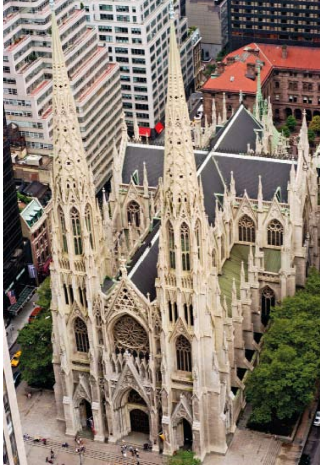
ABOVE Clad in Tuckahoe marble and with spires rising 100 metres from street level, St Patrick's Cathedral in New York is the largest decorated Gothic-Revival Catholic cathedral in North America.
